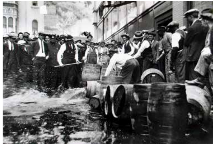
Deputies pour illegal liquor into the street.
